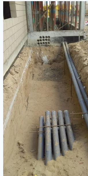
Buried pipework
