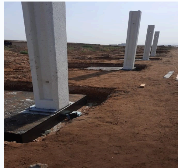
A precast boundary wall going up
