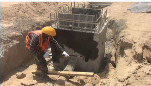
Trenching and drainage
