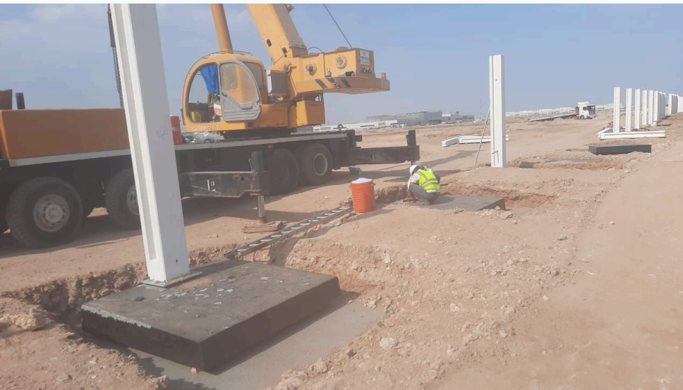
Precast panels, set by crane
