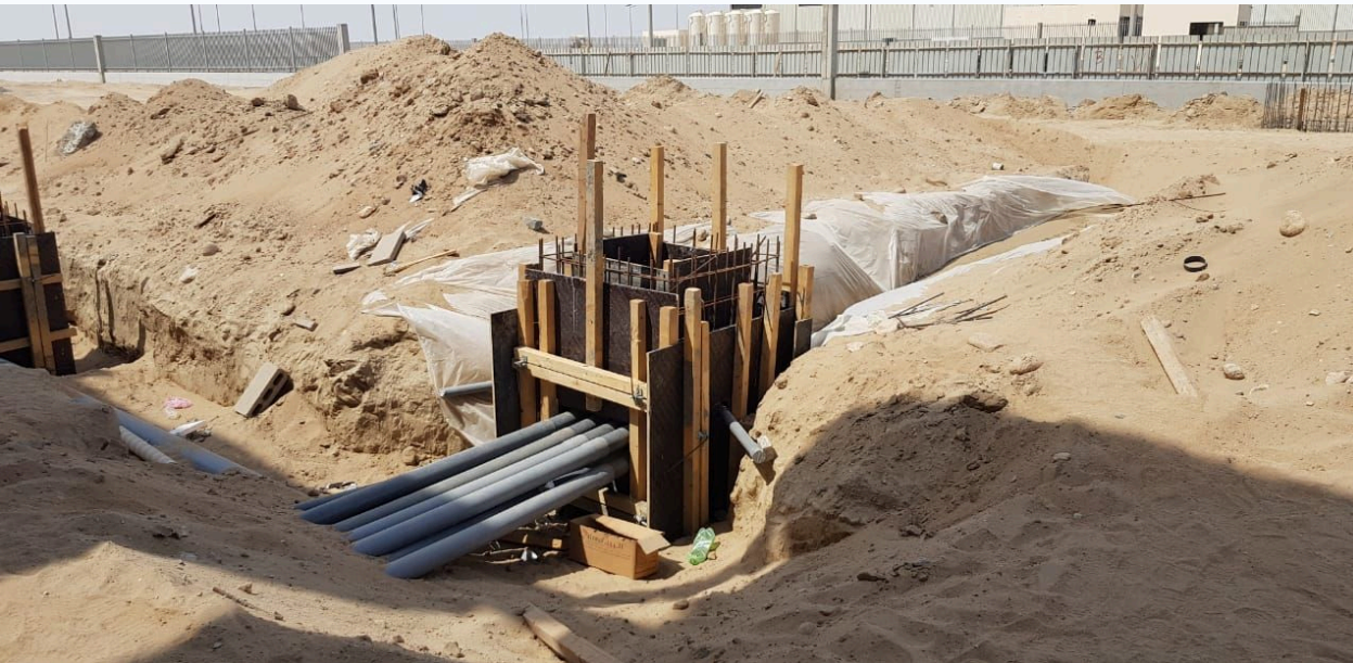
Reinforcement and footings
