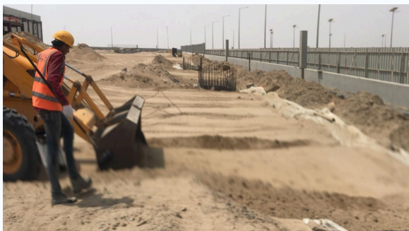
Excavation and earthworks
